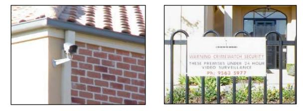
To be most effective, the CCTV system needs to be designed and installed by a qualified person in order that the specification, positioning and lighting requirements are correctly addressed. The system should include provision for recording and be so positioned to reduce the opportunities for the equipment to be vandalised or compromised.
