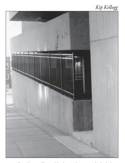
Use of mesh or grilles to block gaps between decks helps to reduce unauthorized access.
