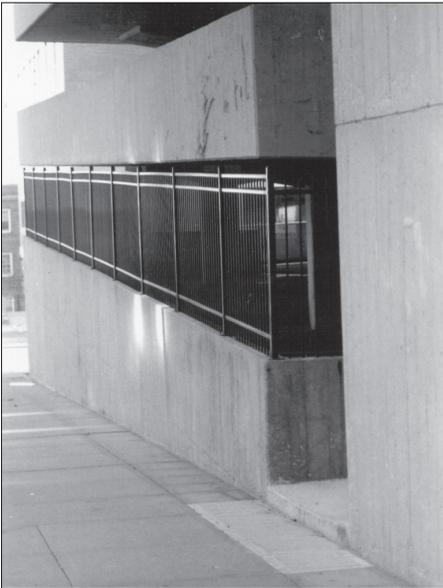
Use of mesh or grilles to block gaps between decks helps to reduce unauthorized access.
